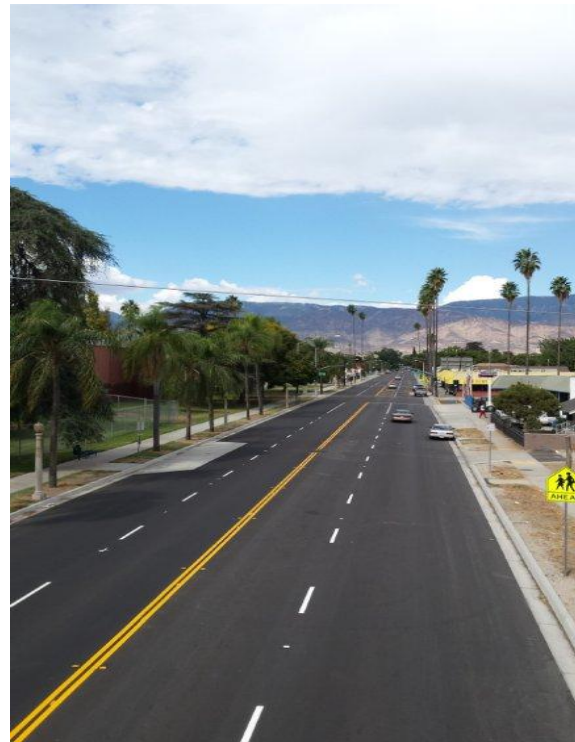
Improved roadway, San Bernardino
