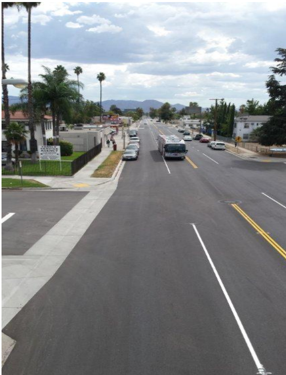
sbX Coach rolling on new roadbed
