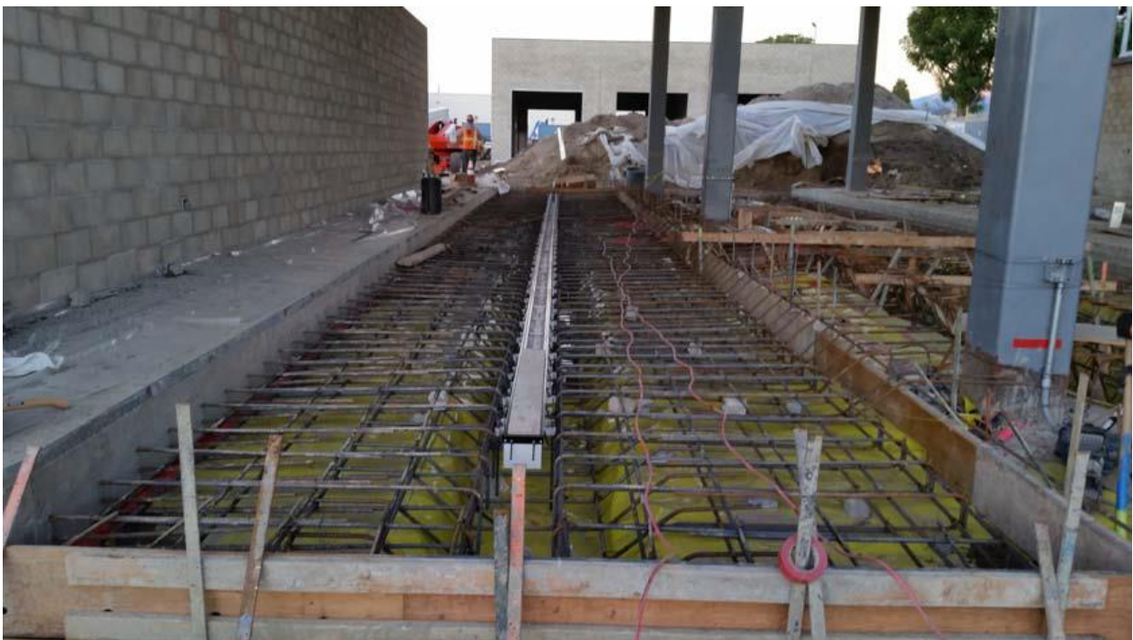
4. BUILDING C – PLACING REINFORCING STEEL FOR TRENCH DRAIN
