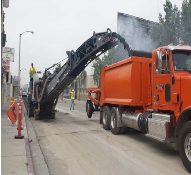
Grinding Asphalt for Repaving
