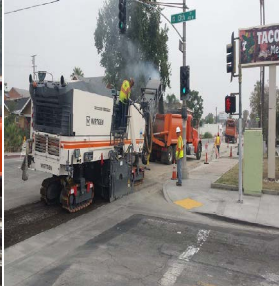
Grinding for Overlay
