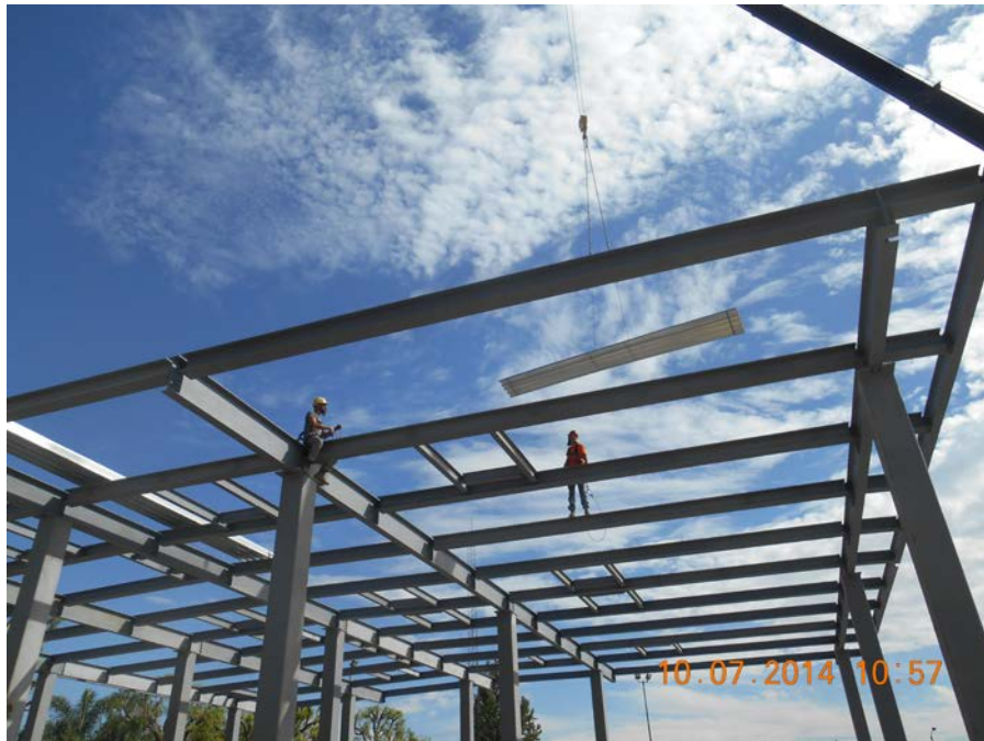
Building C - Receiving and Landing the Roof Decking
