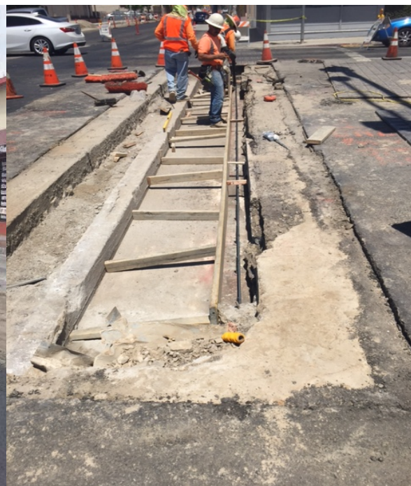
Culvert work at Baseline & E Street
