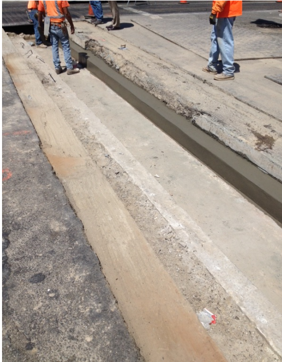
Rebuilt Culvert at Baseline
