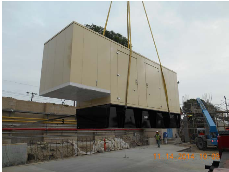
Placement of Generator on the Generator Pad.
