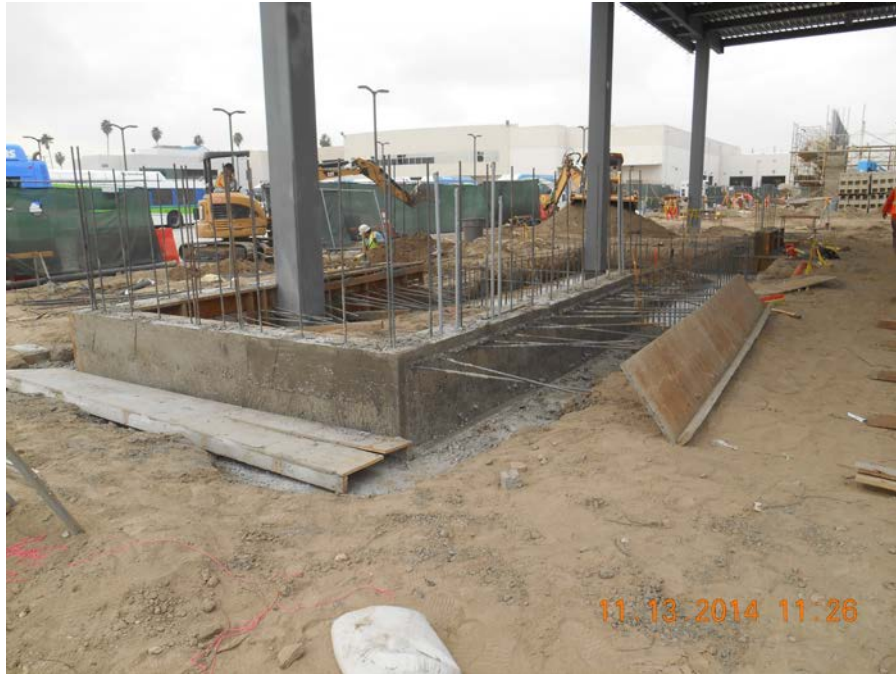
Building C – Removal of forms at stem walls.
