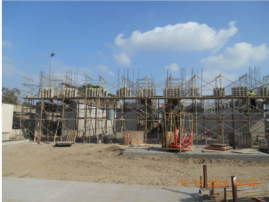
Construction of CMU Wall
