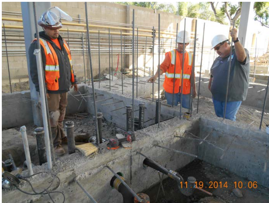
City Inspector signing off the rough-in underground plumbing
