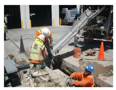
3. Placing concrete in utility trenches (Compressed Air and Cold Water) from Building A to Building C.
