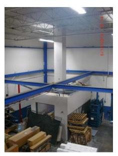
1. Battery Room drywall and shaft is complete in Building A.
