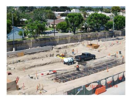
4. Placing reinforcing steel for Inspection Pit, Sewer Ejector Pit, Reclamation Pit and Chassis Wash at Building B.
