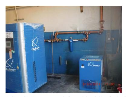
2. New Quincy Air Compressors (2nd out of 2 units) set in the Air Compressor room at Building A.
