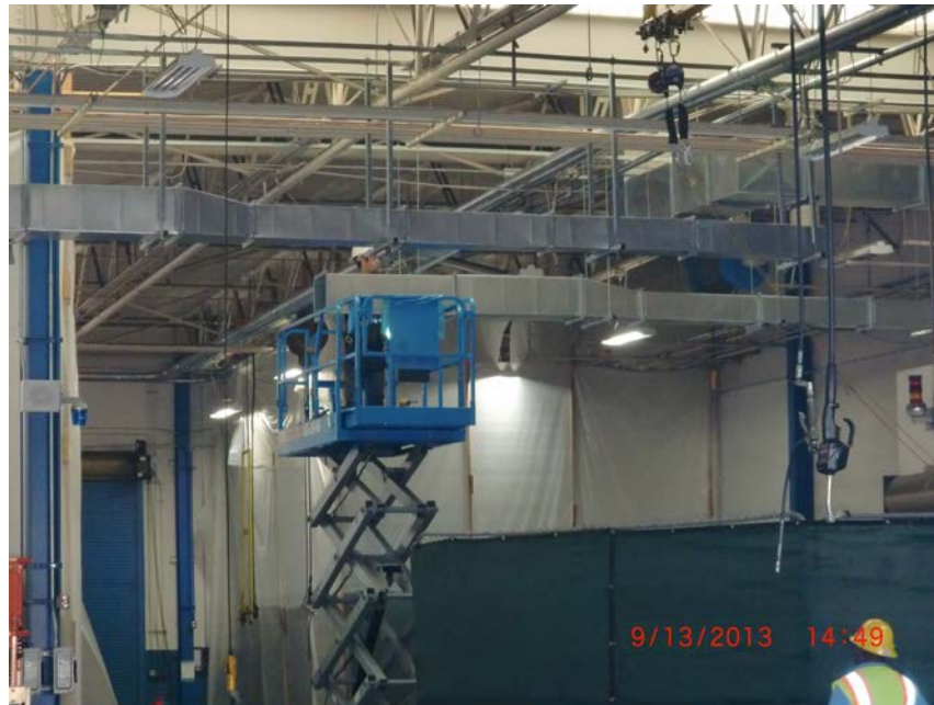
1. Contractor installing HVAC in Maintenance Facility (Building A).
