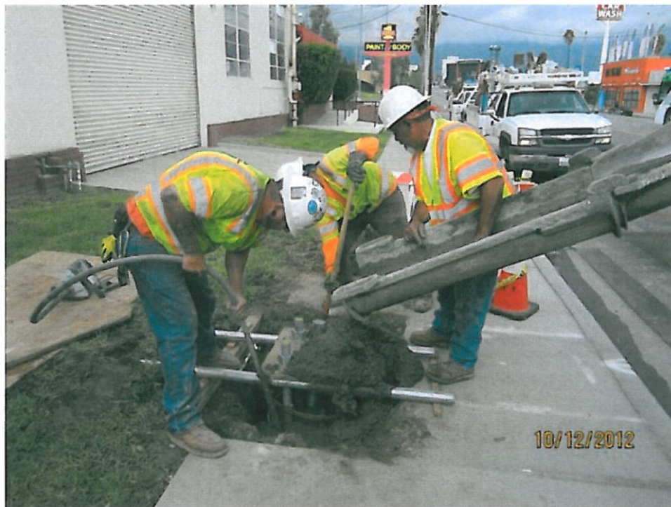
2. E Street – Pouring concrete for traffic signal foundation at the northwest corner of Valley.
