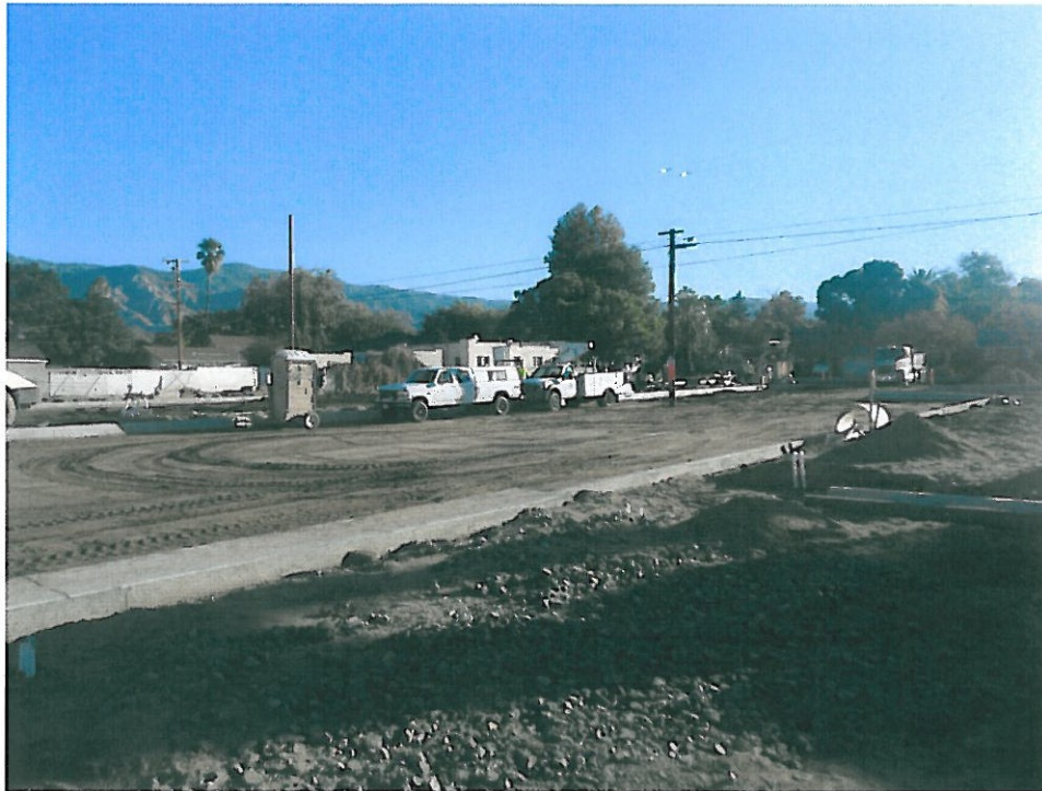
5. Marshall Station (West) – Performing subgrading work.
