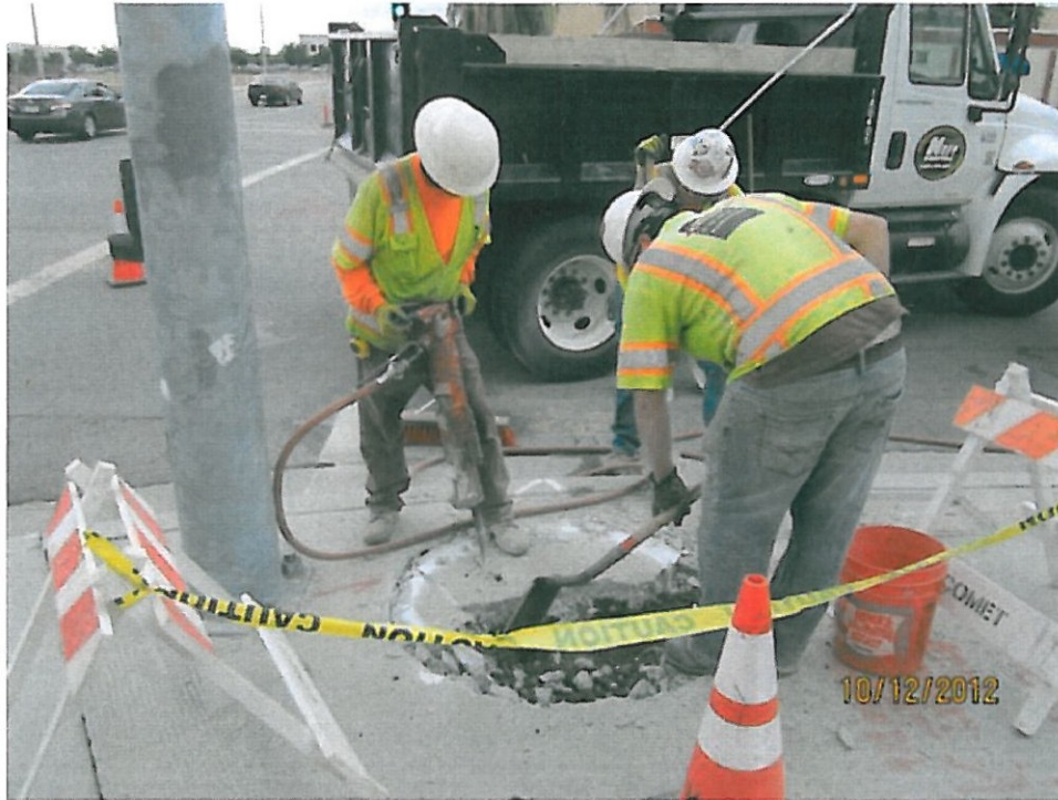
1_ E Street- Potholing for utilities at the northeast corner of Rialto.
