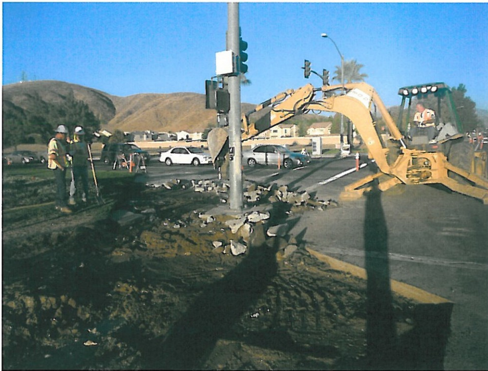
6. Shandin Hills (South) – Demolition and removal of existing asphalt.
