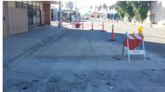
Water Line Trench Patch
