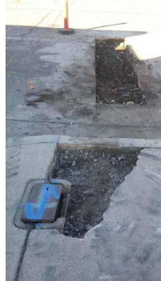
Water Line Trench at Meter
