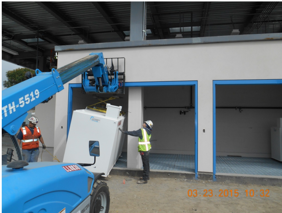
3. BUILDING C – INSTALLING LUBE CUBE TANK
