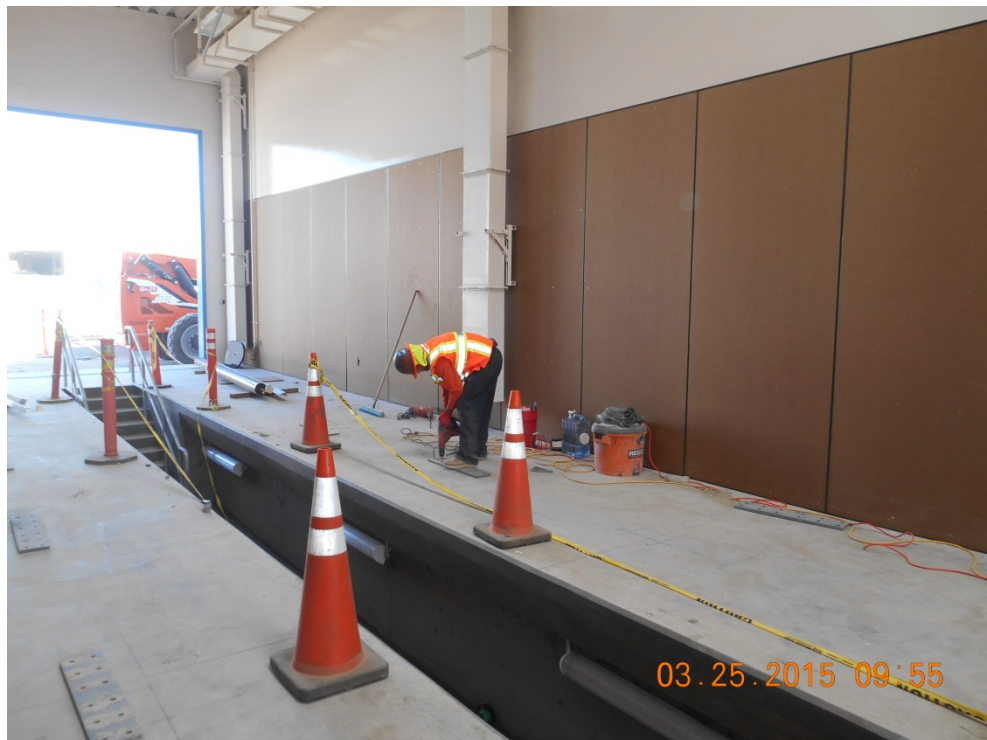
4. BUILDING B – DRILLING FOR WEDGE ANCHORS AT INSPECTION PIT GUIDE RAILS
