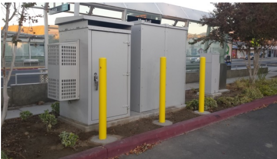
Item #149: Bollards in Front of Electrical Equip.
