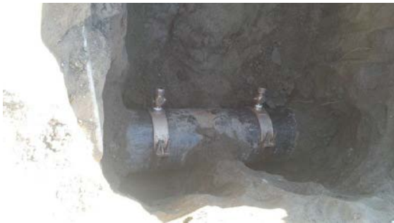
Water Line Connection at Main
