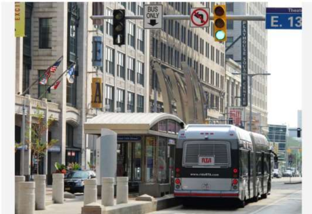
Cleveland's Healthline runs on median-aligned bus-exclusive right-of-way. Photo: ITDP
