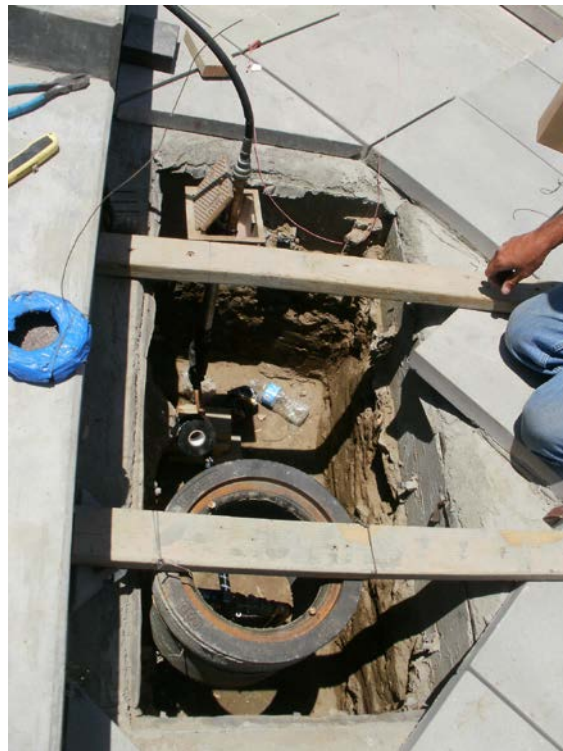
2. Connecting a hose bib to the potable water line at Highland Avenue and E Street.
