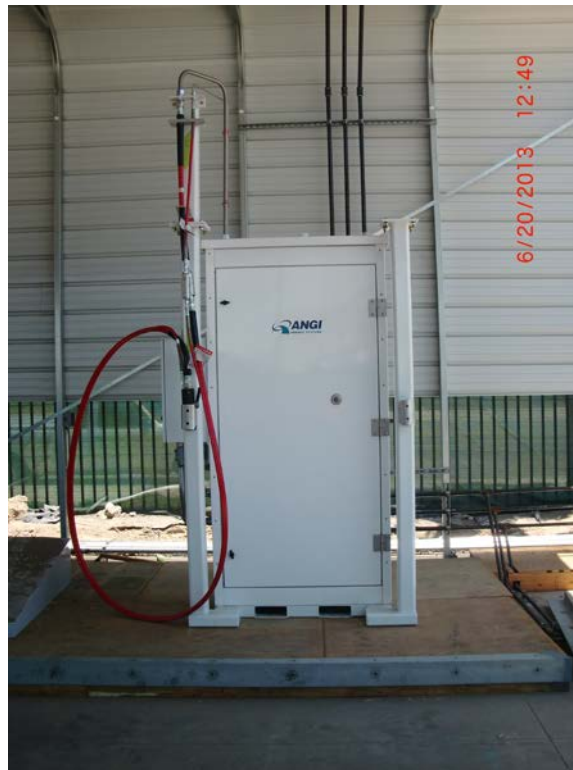
2. CNG Dispensers are installed at the temporary fuel island.
