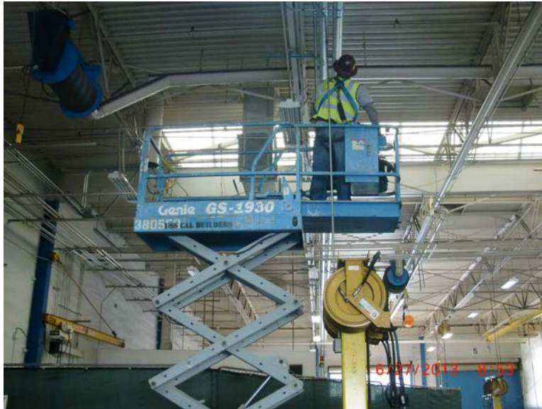
1. Building A overhead conduit installation.
