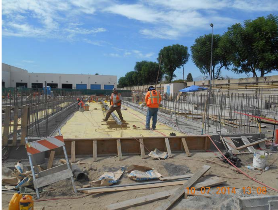
Building B - Installation of Drains at Bus Wash Bay
