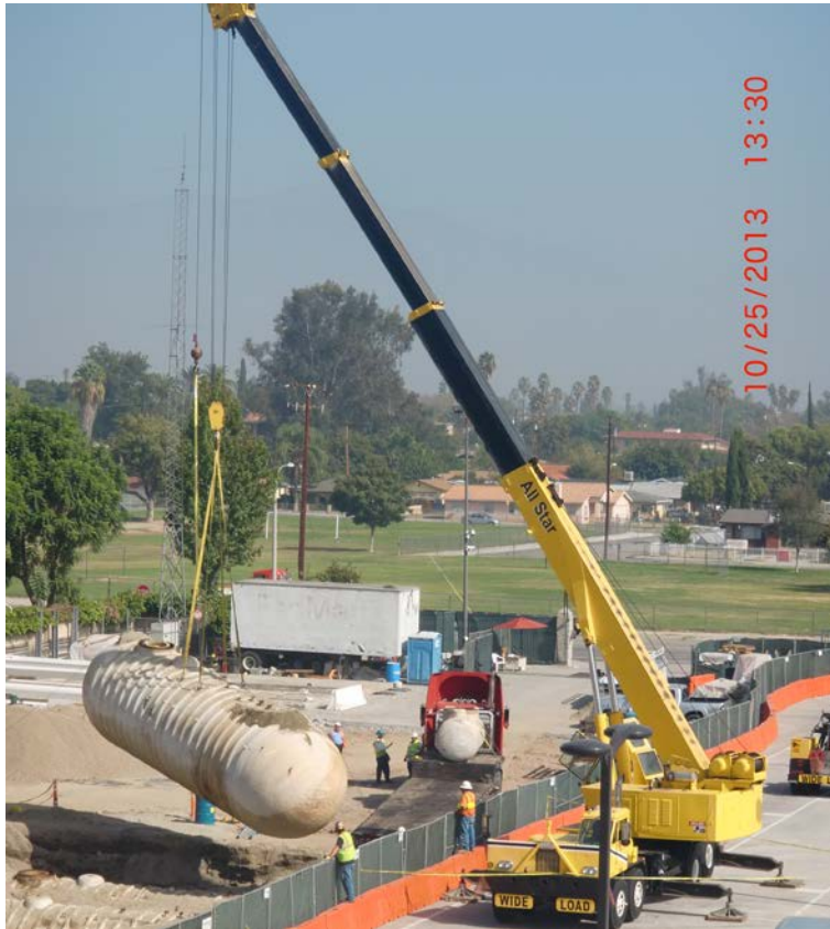
1. Removal of the Underground Storage Tanks (UST)
