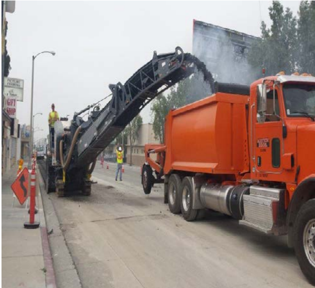
Grinding Asphalt for Repaving
