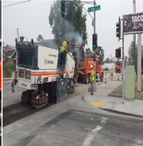
Grinding for Overlay
