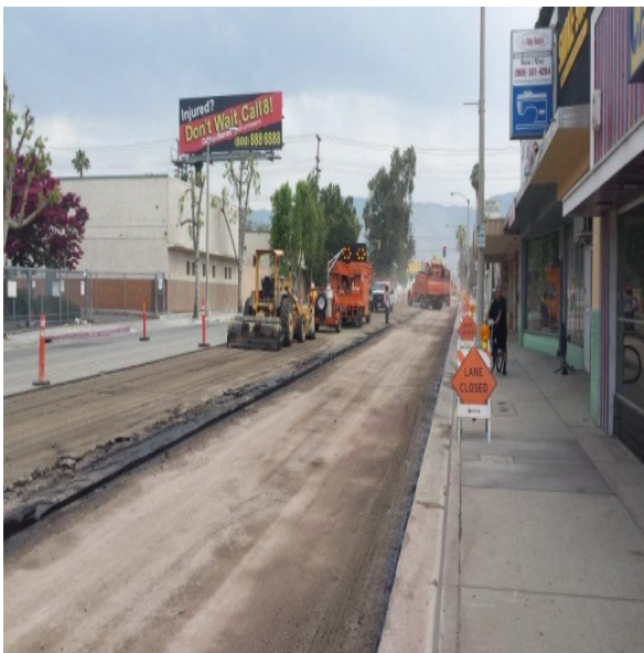
Grind and compaction on E Street
