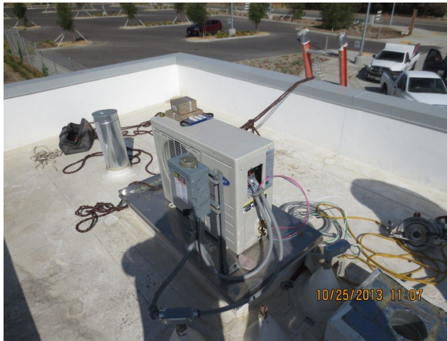
2. Installation of electrical disconnect for HVAC on roof of Restroom at Palm and Kendall station/park and ride location.
