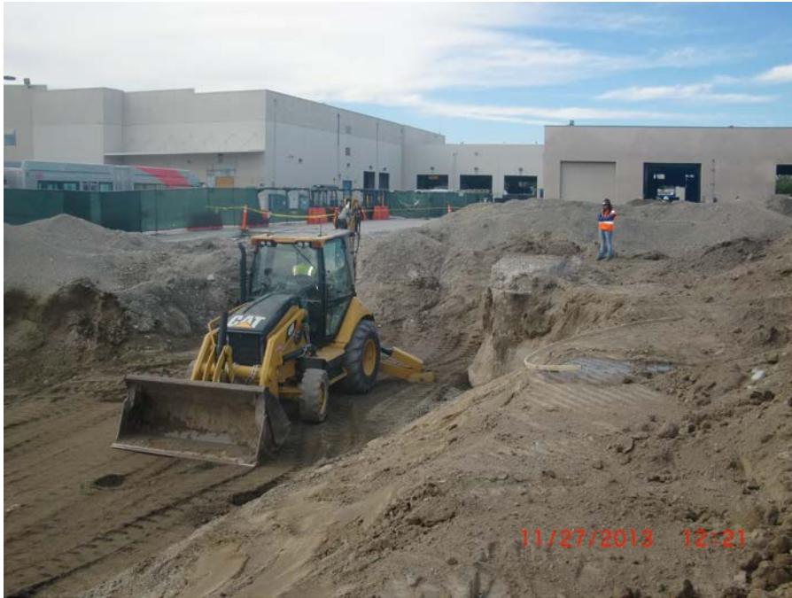
3. Backfill and Compaction of Underground Storage Tank (UST) Excavation.
