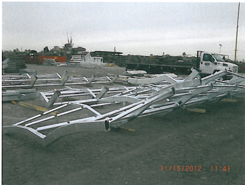
4. Completed Station's canopy steel, (ready for shipping) in the fabrication shop in Arizona.
