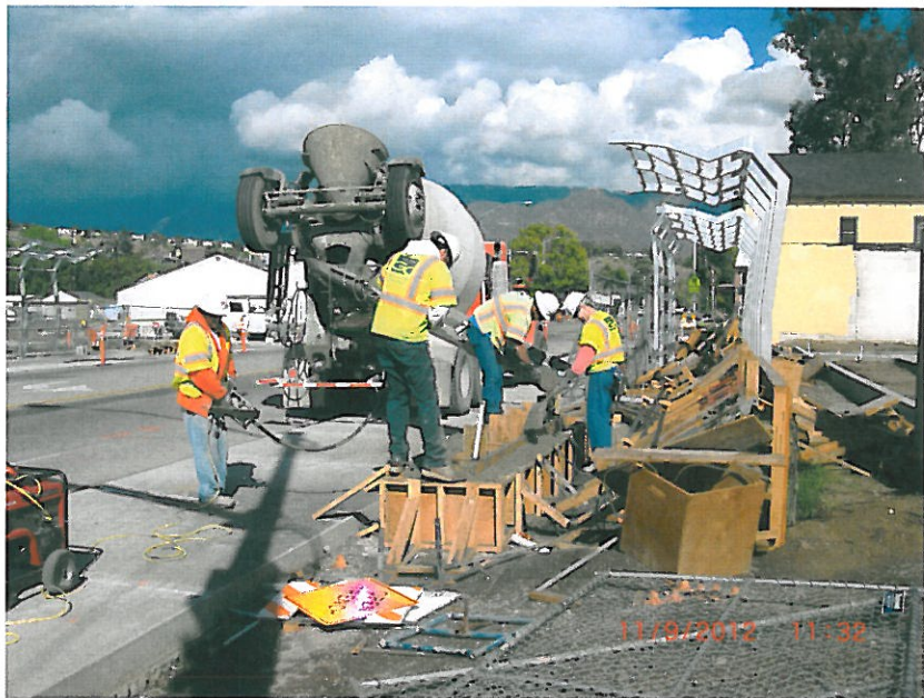
6. E Street & Marshall Station – Pouring planter walls
