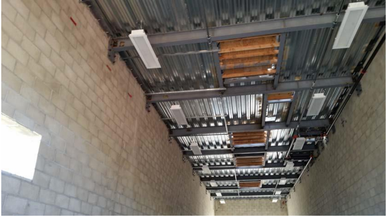
1. BLDG B PREPING SUPPORTS FOR AIR DUCTS
