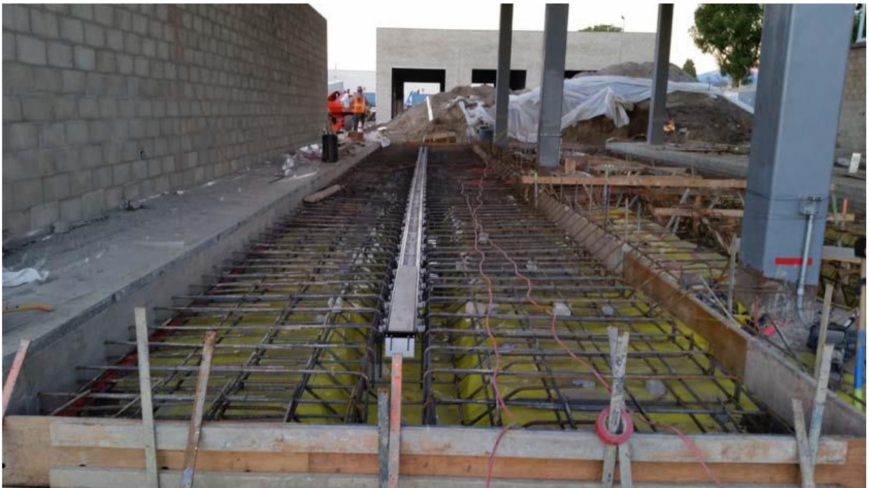
4. BUILDING C – PLACING REINFORCING STEEL FOR TRENCH DRAIN
