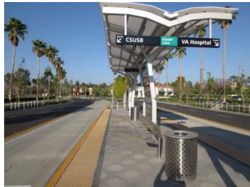
BRT station on sbX line.
