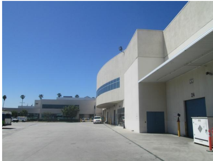
Figure 2-4. Omnitrans East Valley Facility
