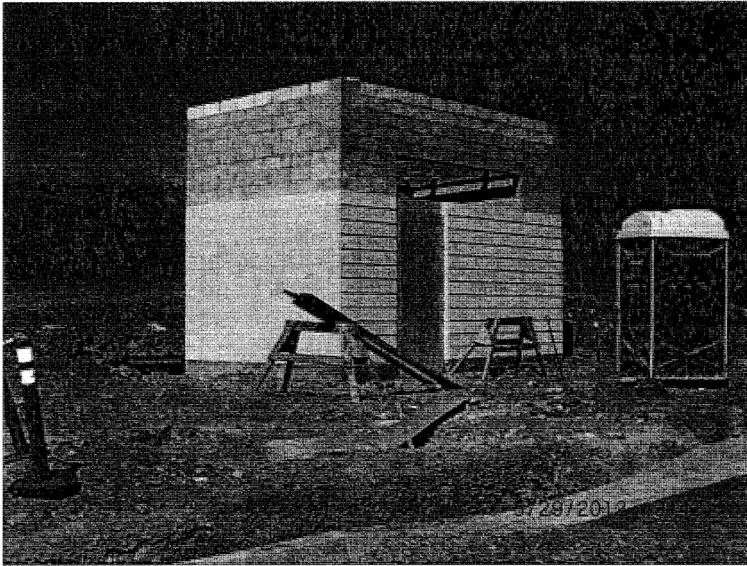
Kendall/Palm – Erected CMU walls for bus driver restroom.
