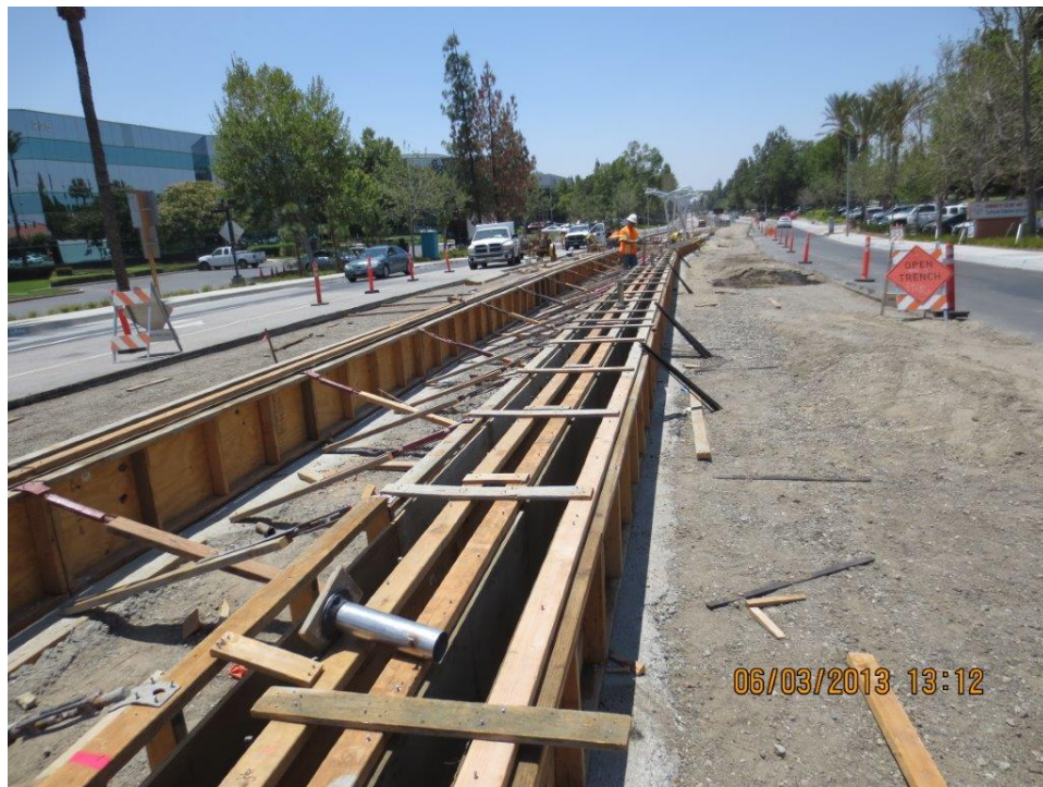
2. Installing Lighted Bollard Imbedded Supports (Typical Project Wide)
