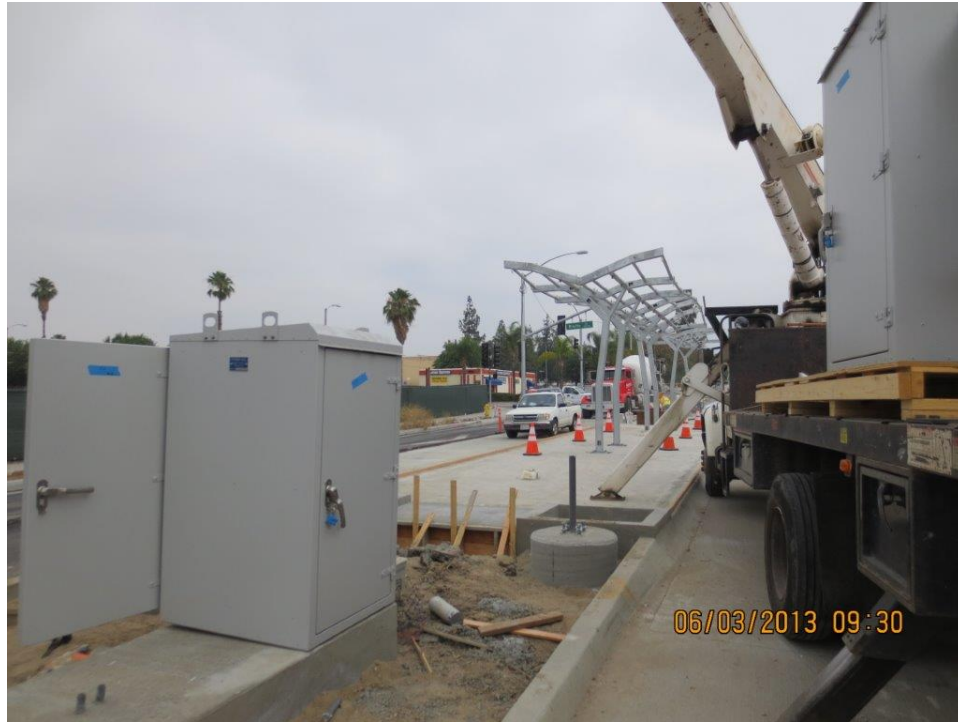
1. Installing Communications Cabinets (Typical Project Wide)
