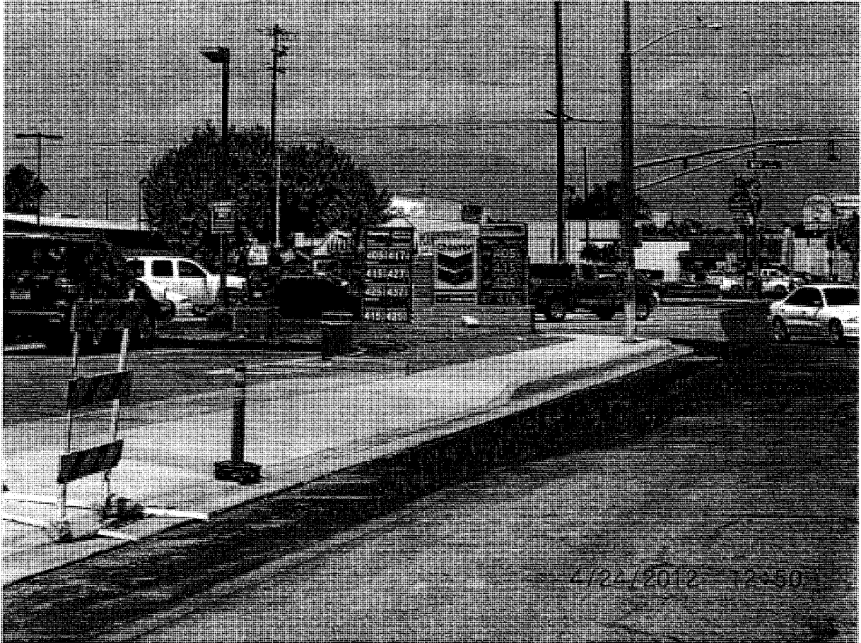
New curb, gutter, driveway & sidewalk and relocated signal pole at SW corner of E Street & Inland Center Drive looking north
