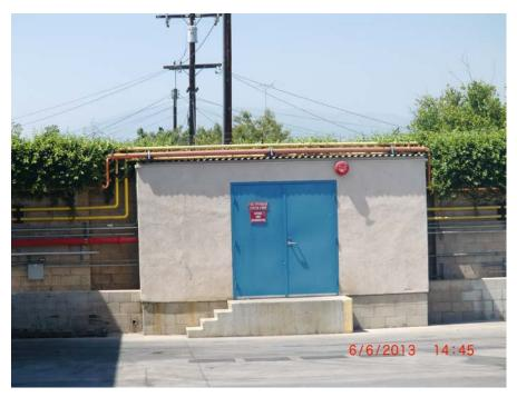
1. Contractor installing the Facility Distribution 4" copper Water Line along the North Site CMU wall and above the existing Fire Pump Enclosure.
