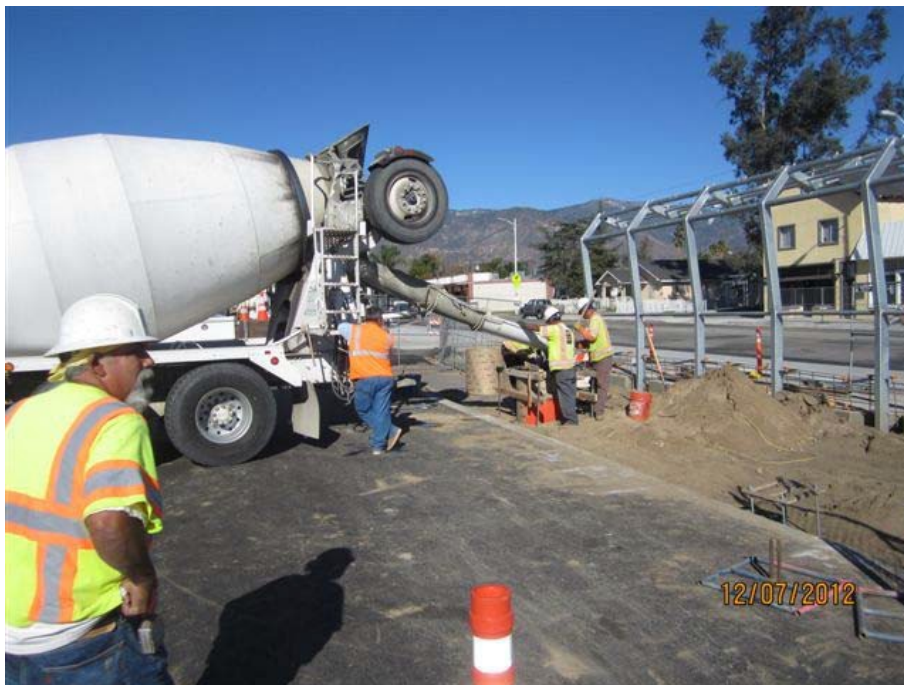
2. Marshall West Park-N-Ride - Form and pour solar lighting foundation.
