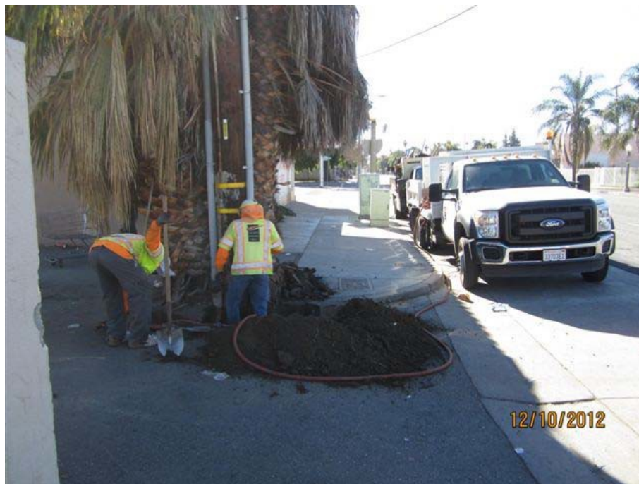
6. E Street - Pothole for utilities.
