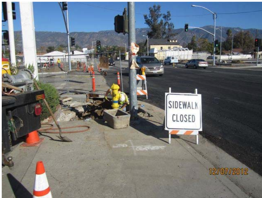
4. E Street - Termination of traffic signal crossing at Marshall.
