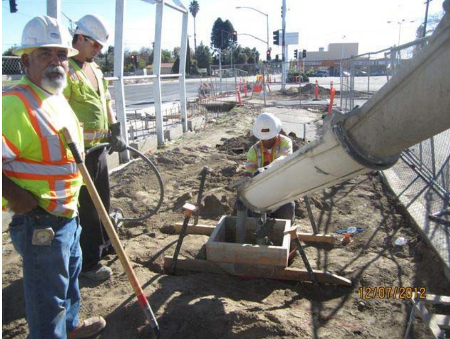
1. Marshall West Park-N-Ride - Form and pour meter pedestal foundation.
