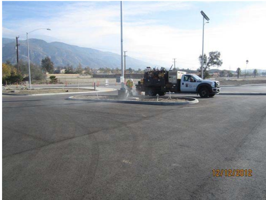
5. Kendall/Palm Park-N-Ride - Applying masonry finish to raised pole foundations.
