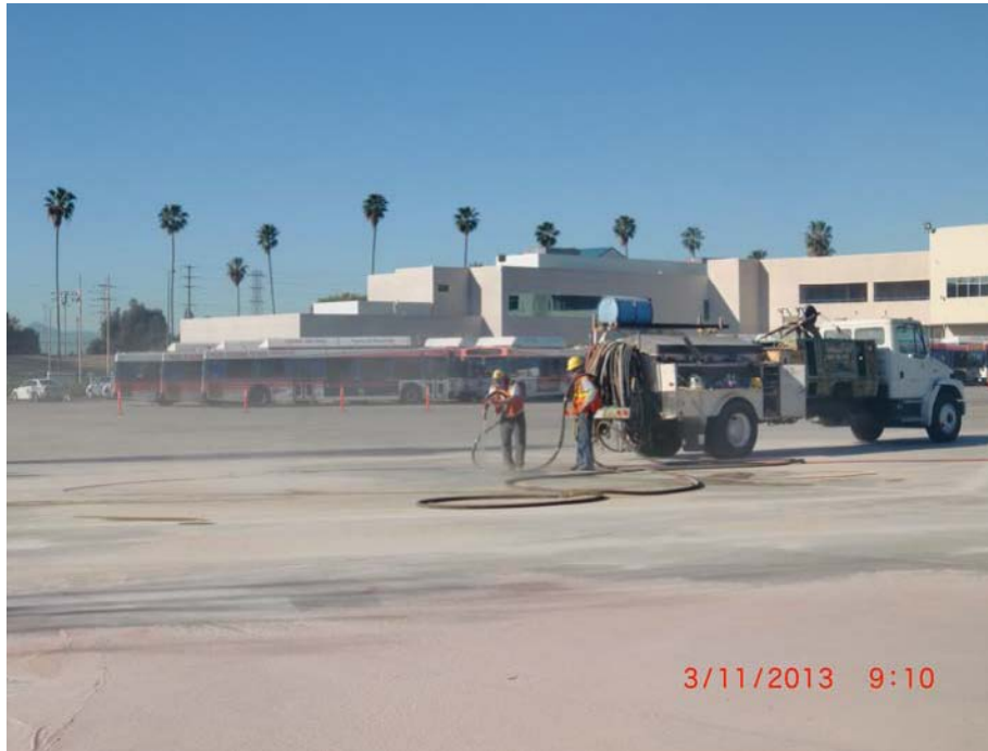
1. Sand blasting of existing parking lot striping.
