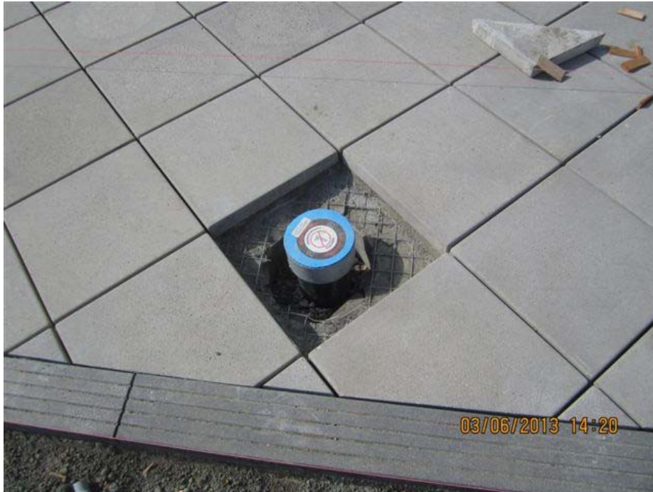
1. Recessed platform light installation.
