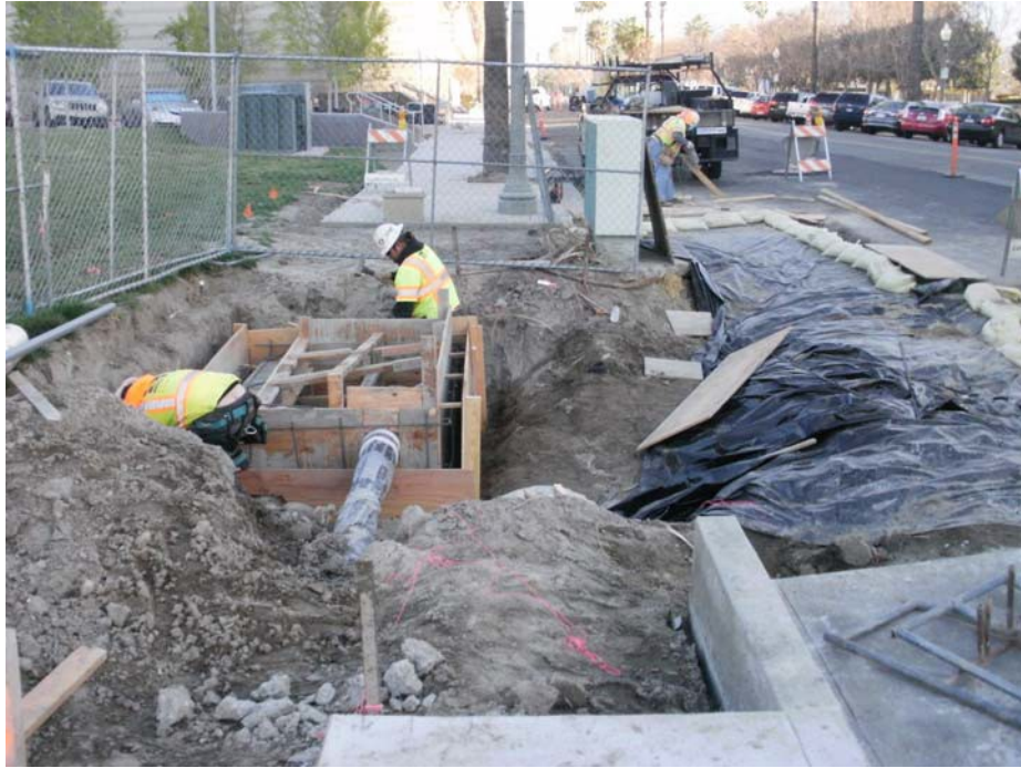
3. E Street at 4thStreet - Geothermal formwork vault
