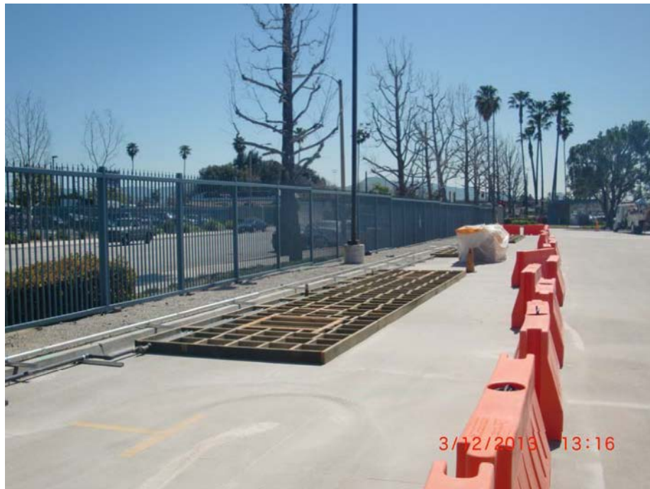
2. Frame work for the temporary fuel island platform.
