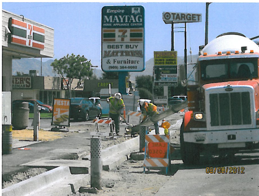
4. E Street, North of Orange Show – Street light foundation.
