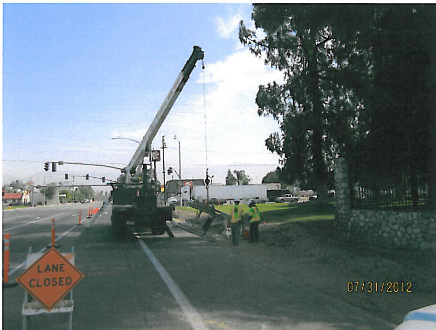
6. Pole setting operation northbound E Street/Mill Street.
