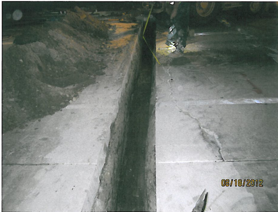
5. Excavate trench for traffic signal conduit run # 8 across south bound at Waterman/Hospitality.
