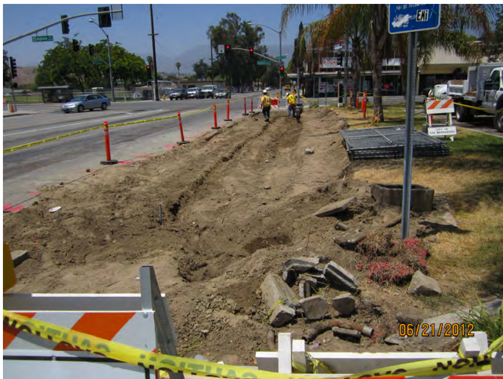
Highland Station North – Backfill and compact electrical trench.
