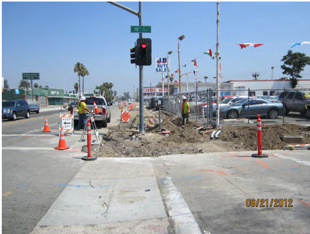
10 th Street and E Street – Excavating trench for traffic signal conduit.
