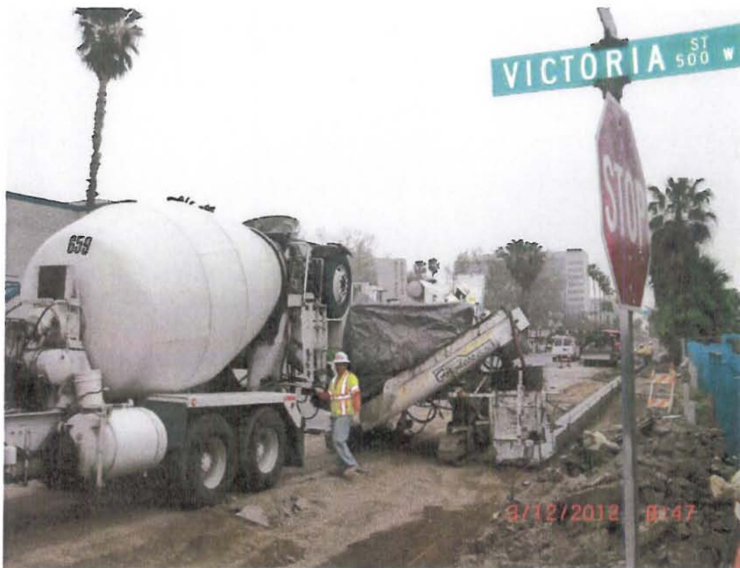
Placement of Curb & Gutter on E Street at Victoria Street
