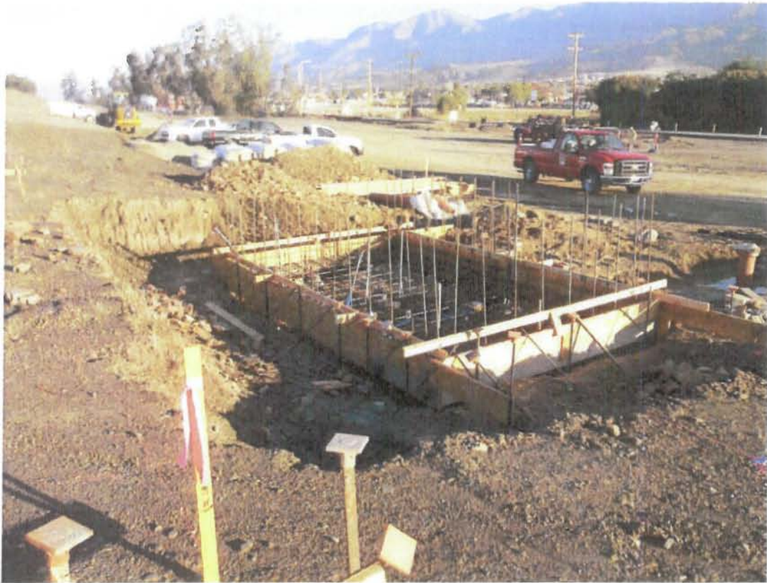
Formwork and reinforcement for the restroom slab on grade at the Palm/Kendall Park & Ride
