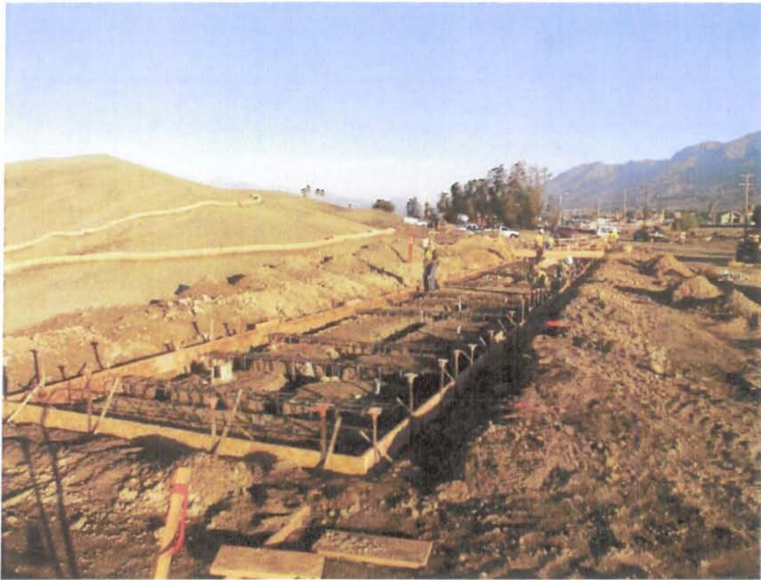
Formwork for Bus Platform at Palm/Kendall Park & Ride
