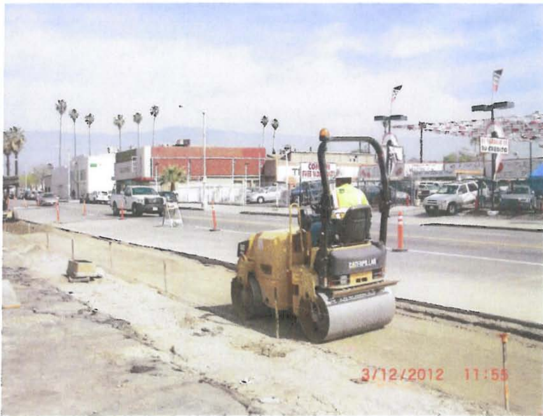
Compaction of sub-grade on E Street between 9 th and 10 th Streets
