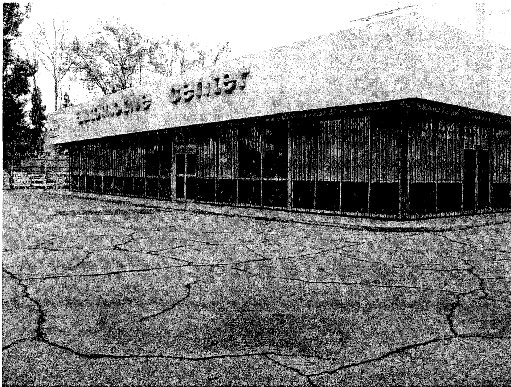
Griffith/Comet Project Field Office
