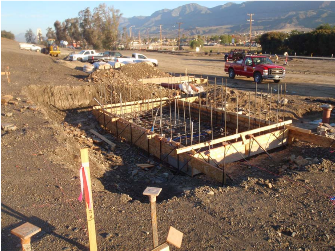
Formwork and reinforcement for the restroom slab on grade at the Palm/Kendall Park & Ride
