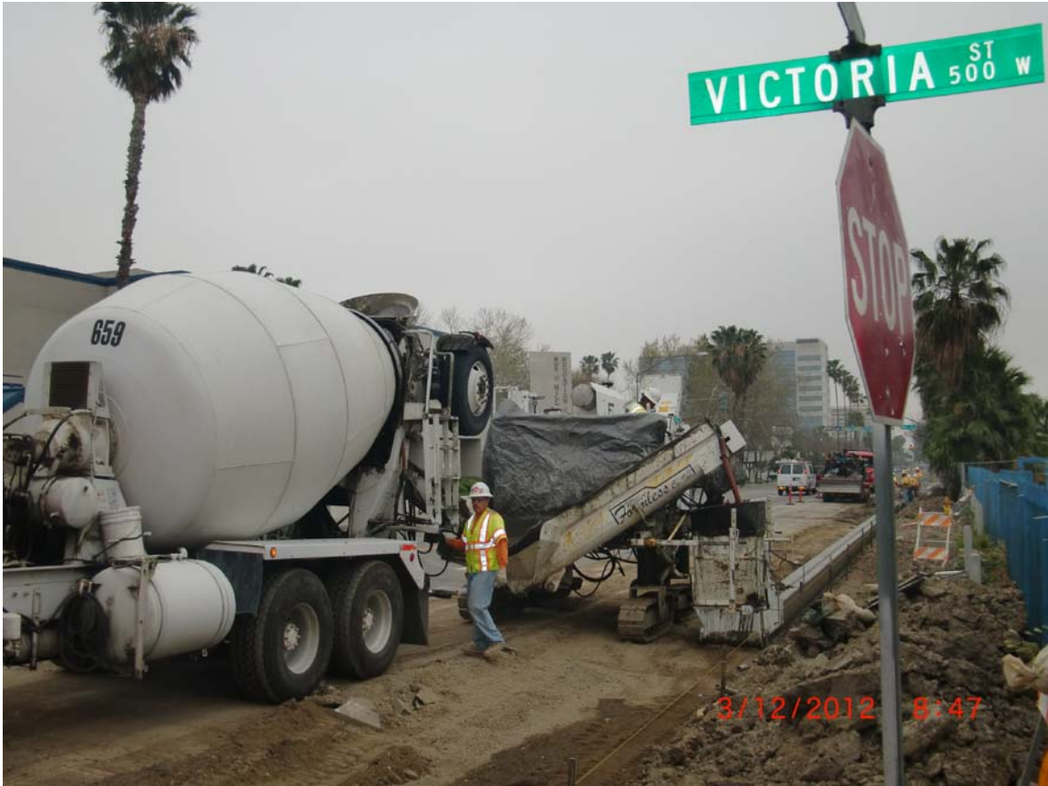
Placement of Curb & Gutter on E Street at Victoria Street
