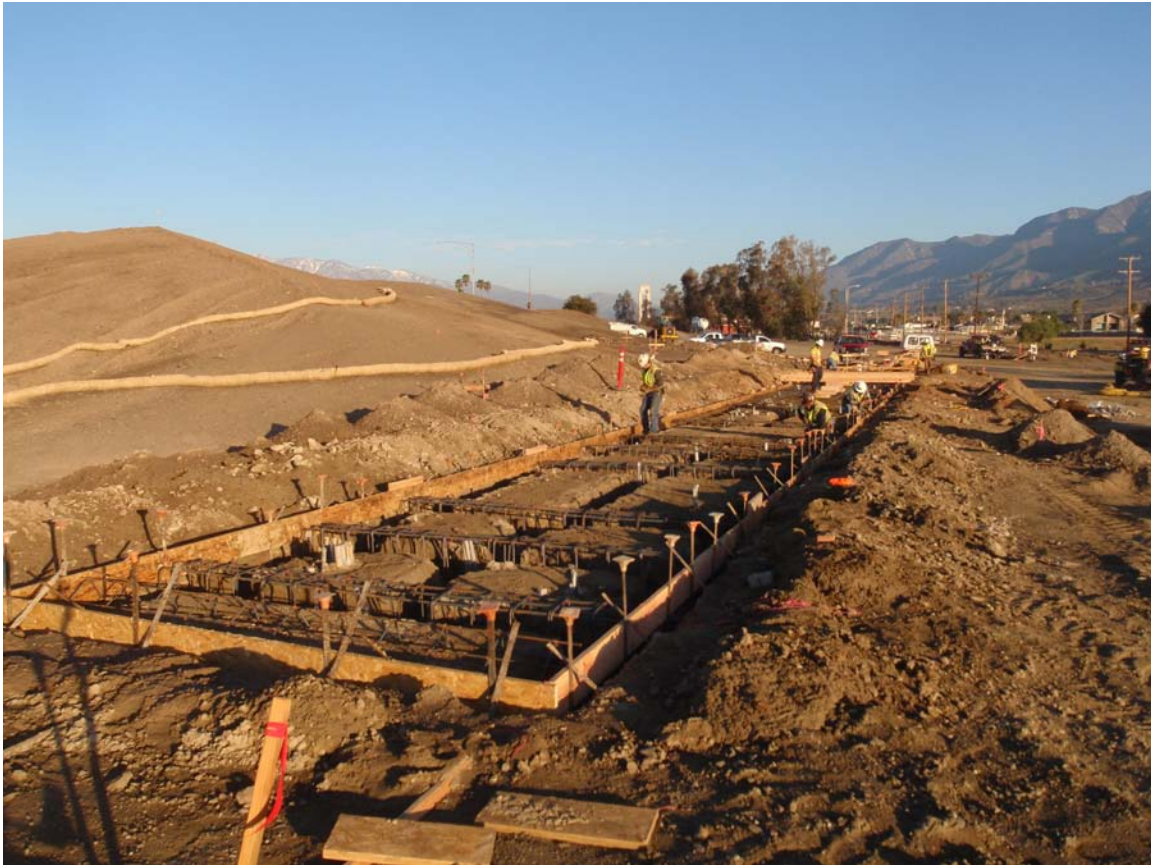
Formwork for Bus Platform at Palm/Kendall Park & Ride
