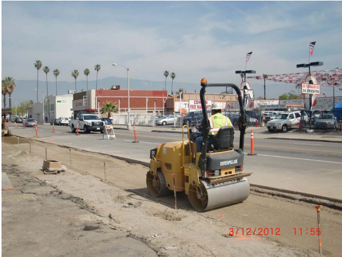
Compaction of sub-grade on E Street between 9 th and 10 th Streets
