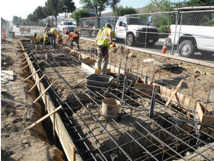
3. Little Mountain – West side station platform foundation.
