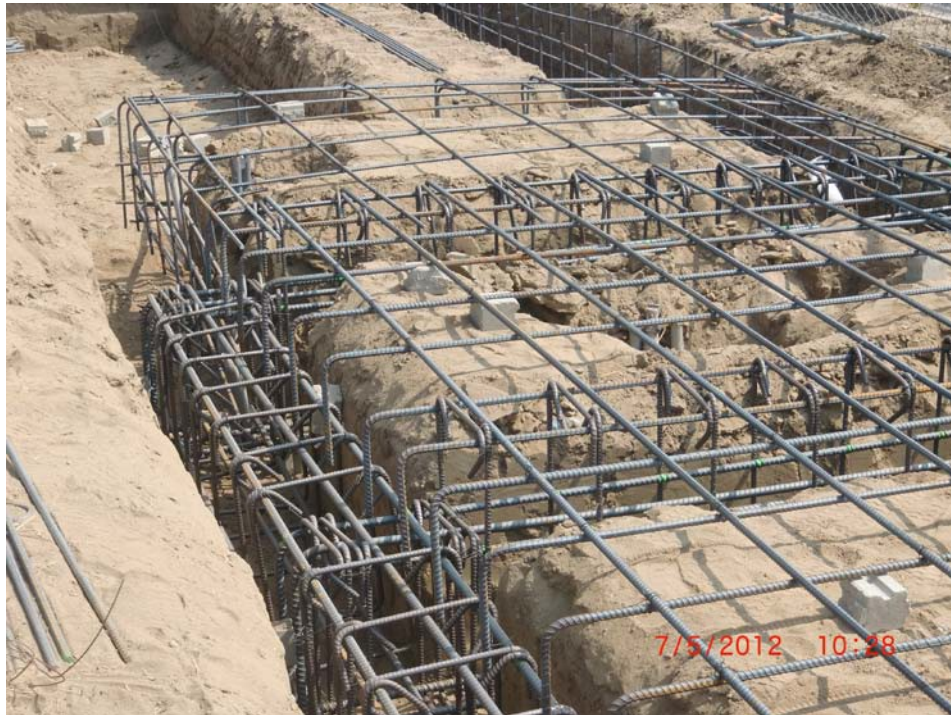
5. E Street/ Marshall Station (West) – Reinforcement for bus station platform.
