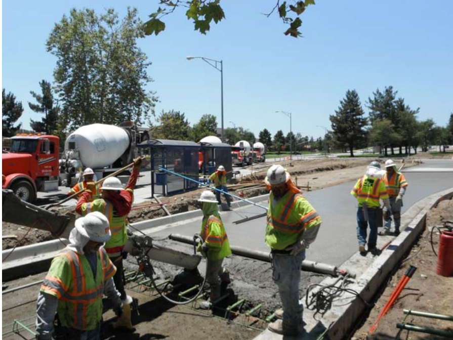
1. CSUSB Station – Bus loop route entrance; 10" PCC paving.
