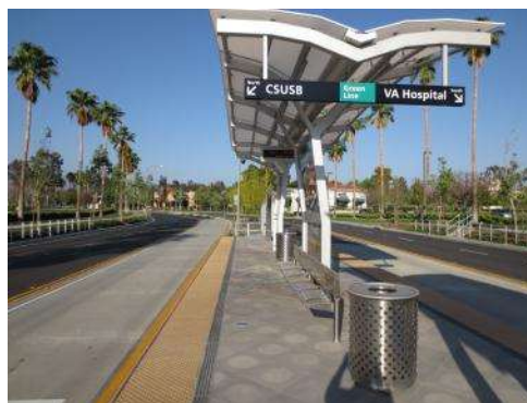
BRT station on sbX line.
