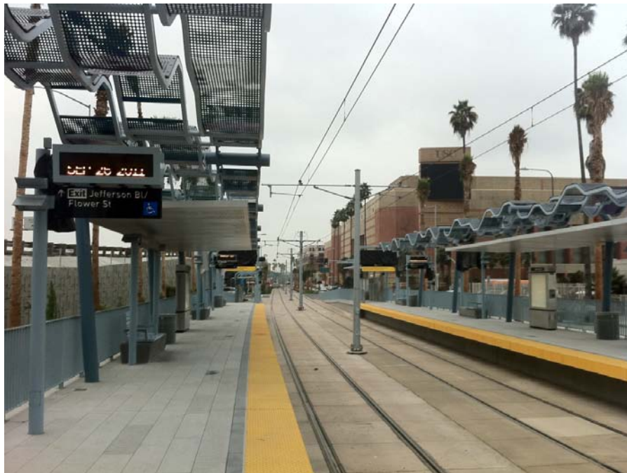
Figure 3-8: Light Rail Station with Overhead Catenary System
