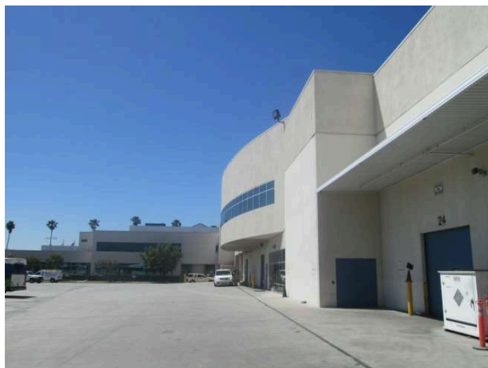
Figure A- 6. Omnitrans East Valley Facility
