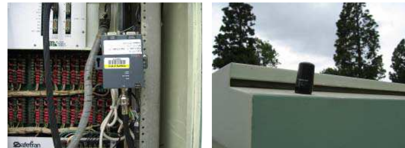
Figure 11-8: Terminal Server and Cabinet-Mounted Antenna
