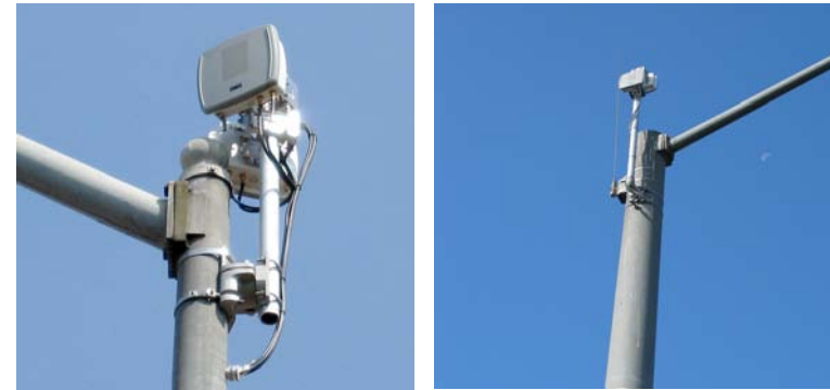
Figure 11-6: Typical WLAN AP/Bridge Equipment Installations
