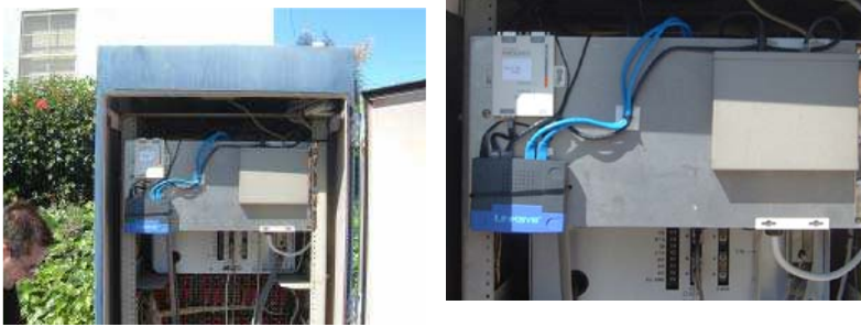
Figure 11-7: AP/Bridge Equipment Panel In Type 332 Traffic Cabinet
