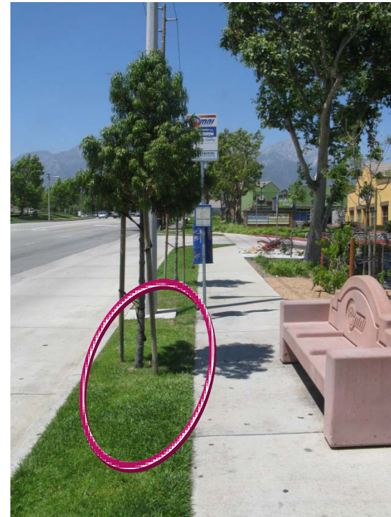
Figure 6-1: Example of a bus stop without an ADA landing area, where passengers do not have an accessible path to the bus door.
