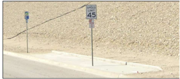
No curb connection to the sidewalk. No clear path to ramps or intersections. There are no sidewalks.
