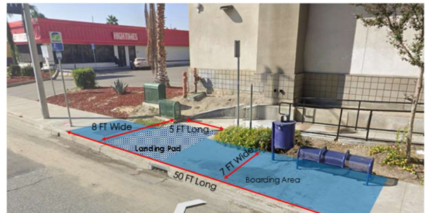
BASIC: Meets all the requirements. The landing pad is at a minimum of 8' x 5' but is not immediately adjacent to the bus stop pole.
