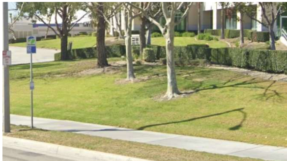
There is no landing pad or boarding area. No curb connection to the sidewalk.
