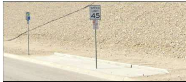
No curb connection to the sidewalk. No clear path to ramps or intersections. There are no sidewalks.
