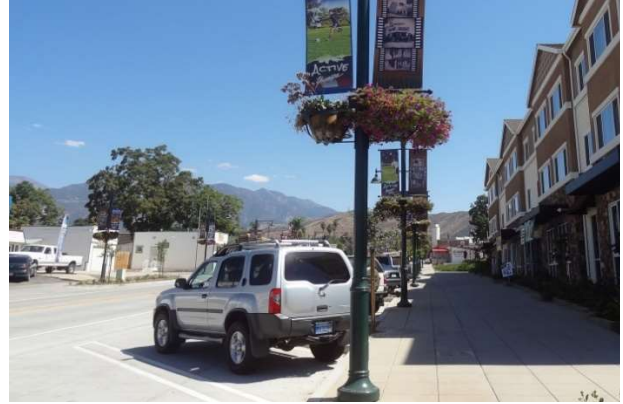
Figure 1-11: Angled parking protects pedestrians from moving traffic in Yucaipa's mixed-use Old Town District
