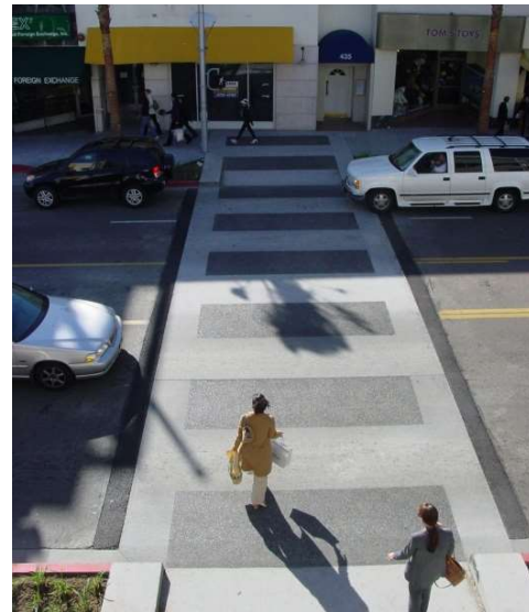
Figure 1-22: High visibility crosswalks increase pedestrian safety.
