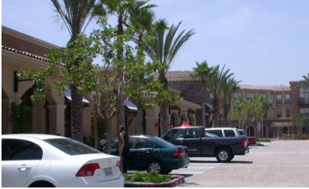
Figure 1-7: A mixed-use area with landscaped pedestrian pathways and textured paving of parking areas, Rancho Cucamonga, CA
